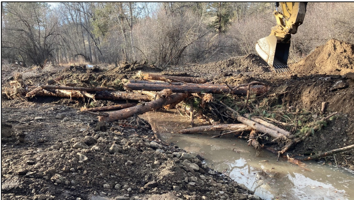
SIDE CHANNEL 5 POOL AND LARGE WOOD STRUCTURE
