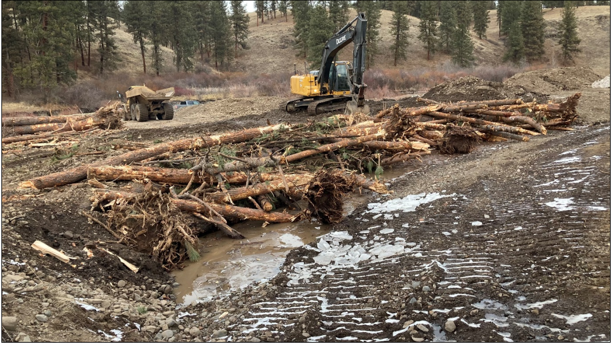
SIDE CHANNEL 5 POOL AND LARGE WOOD STRUCTURE
